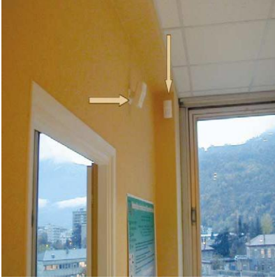
Figure 2. Activity generic sensors (infrared volumetric sensors indicated by arrows).
